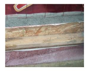
or you can do the mixing by hand. Don't try and use a cement mixer. It won't work. The paint, cement and sand will stick to the inside of the barrel and won't mix with the foam. Because the mix is light, mixing by hand will not be a difficult job. This is not a mix that can be poured, it must be shoveled and packed.
